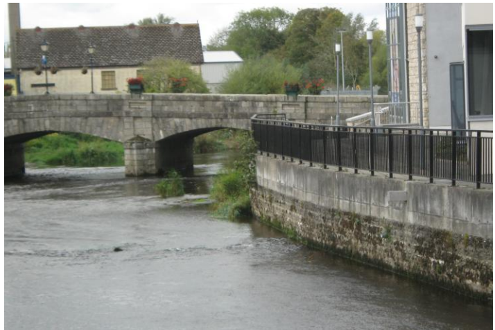
The site where sewage is discharged directly in Tullow.
