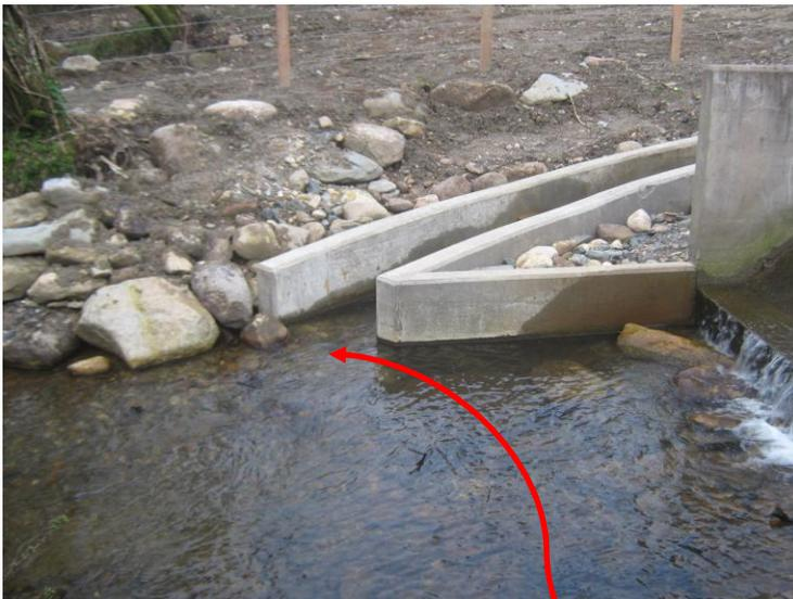
Base of the pass has considerable head (measure of flow) to attract fish, small problems still exist for the larger sea trout and salmon which require greater head of water to be attracted to enter the pass than is currently being created by the flow through the pass
