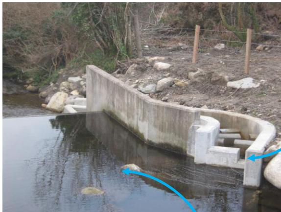
Fish pass consists of successive chambers which appear to have no flow over the cut notch but on close inspection there is a 10 inch square opening on the river bed on each chamber wall at the opposite side to the above water line visible notch, basically each chamber fills from below
